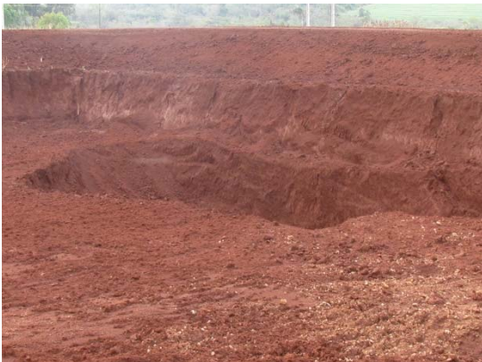
Pit Area with Tailings Sump
