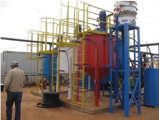
Adjustment Tanks and Sweco Screens
