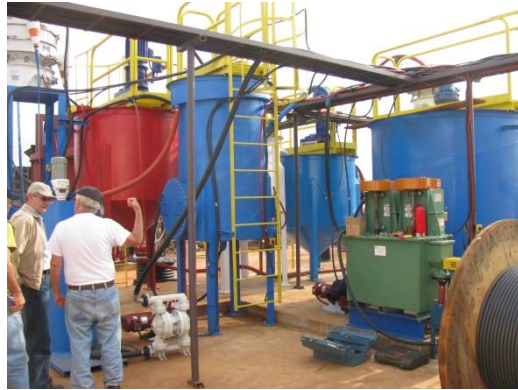
Hydroseparator (red) Tank Elution (blue) Column Attrition Scrubber (green)
