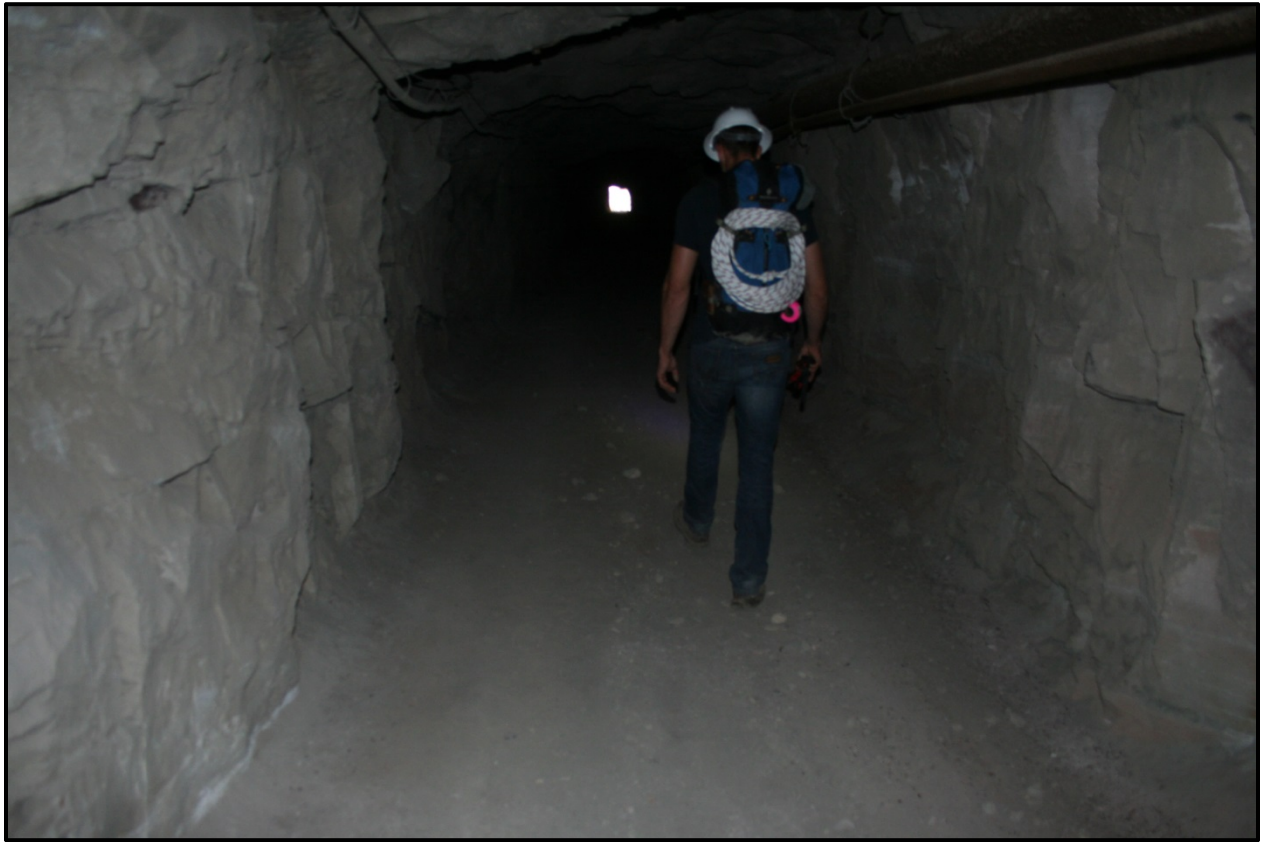
FIGURE 16.3: CONDITION OF BURRO MINE DECLINE
