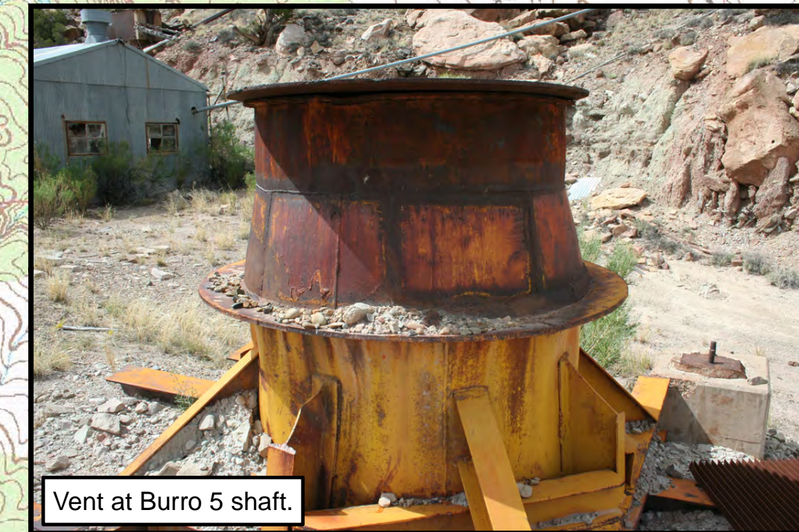
Vent at Burro 5 shaft.
