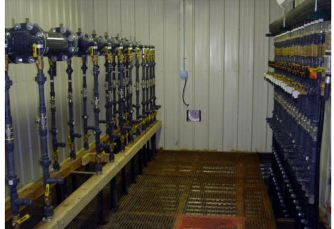
*Inside a “header house.” Many who know how ISR (Solution Mining) operations work compare this to a water treatment plant. The tubes connect to the aquifer from where the uranium is extracted. Right: Water in; water out. Just as you would find at a water treatment facility.*
