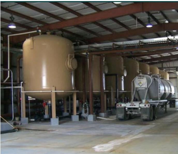
*Each 11.5 ft. ID ion exchange vessel contains 500 Ft<sup>3</sup> resin. Three trains of vessels are installed. Each train consists of two vessels that are operated in series. Upon exiting the 2nd ion exchange vessel, the lixiviate is pressurized by the 2nd booster pump station, refortified with oxygen and injected into the Well Fields.*
