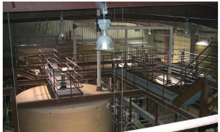
*A three-staged elution circuit is used for uranium concentration that is required for precipitation of a yellowcake product. As an eluate batch advances forward and contacts a new resin bed, the uranium concentration in the batch is increased. Over 90% removal efficiency is achieved in the first elution step.*
