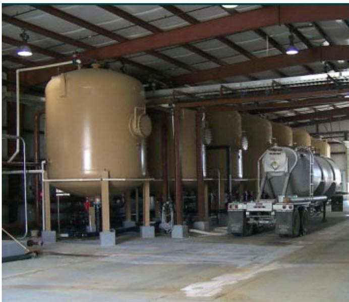
*Each 11.5 ft. ID ion exchange vessel contains 500 Ft<sup>3</sup> resin. Three trains of vessels are installed. Each train consists of two vessels that are operated in series. Upon exiting the 2nd ion exchange vessel, the lixiviate is pressurized by the 2nd booster pump station, reformed with oxygen and injected into the Well Fields.*
