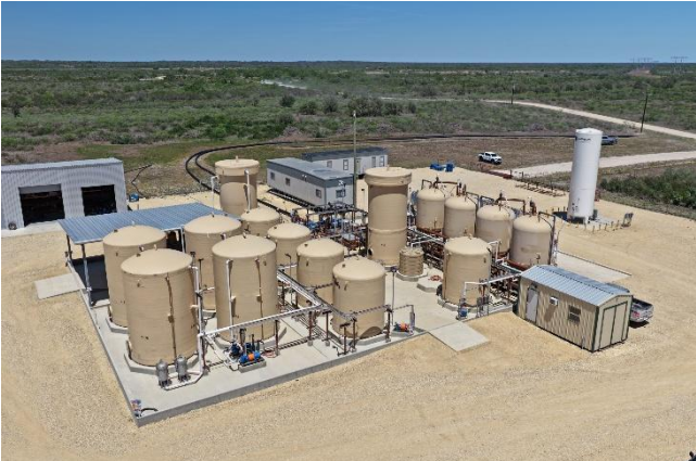
Burke Hollow Satellite Site
