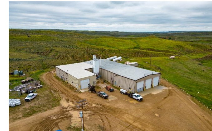
Christensen Ranch Plant Exterior
