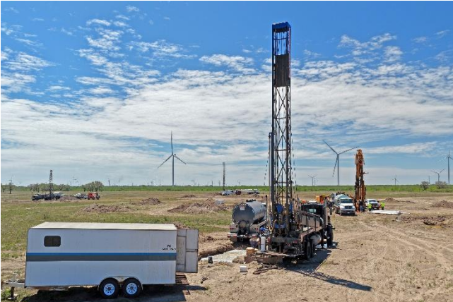
Drill Rig at Burke Hollow
