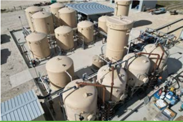
Burke Hollow Satellite Site
