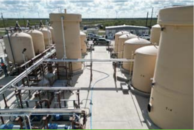
Burke Hollow Satellite Site
