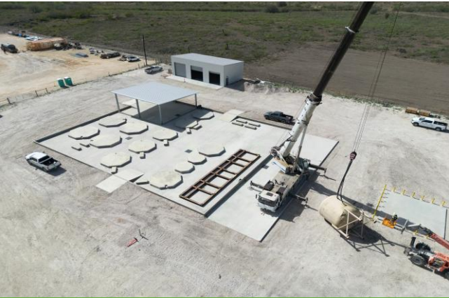
Construction at Burke Hollow
