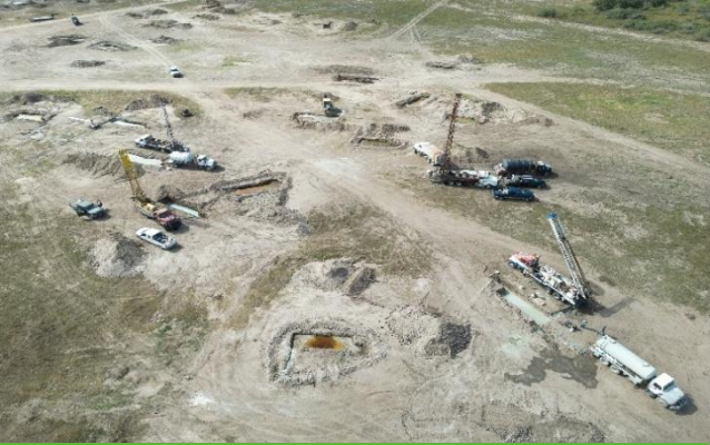
Drilling at Burke Hollow
