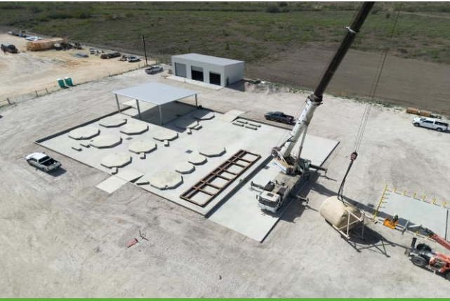
Construction at Burke Hollow
