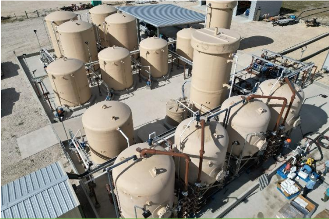
Burke Hollow Satellite Site
