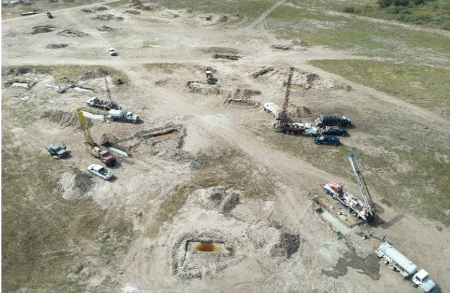
Drilling at Burke Hollow
