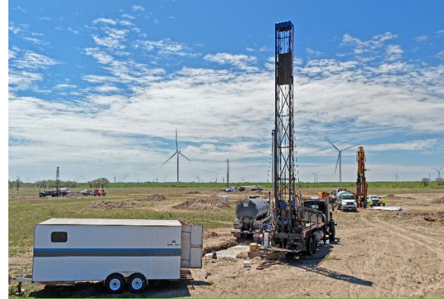
Drill Rig at Burke Hollow
