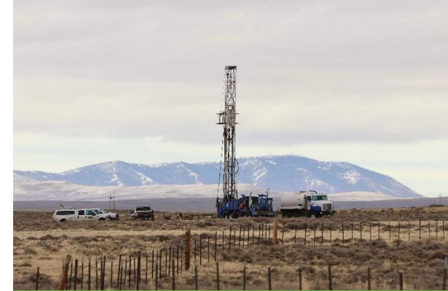
Drill Rig at Sweetwater
